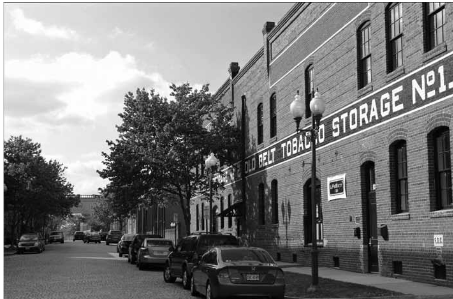
The high-tech computer facility sits inside a refurbished building known as Old Belt No. 1, which was constructed in 1877.
